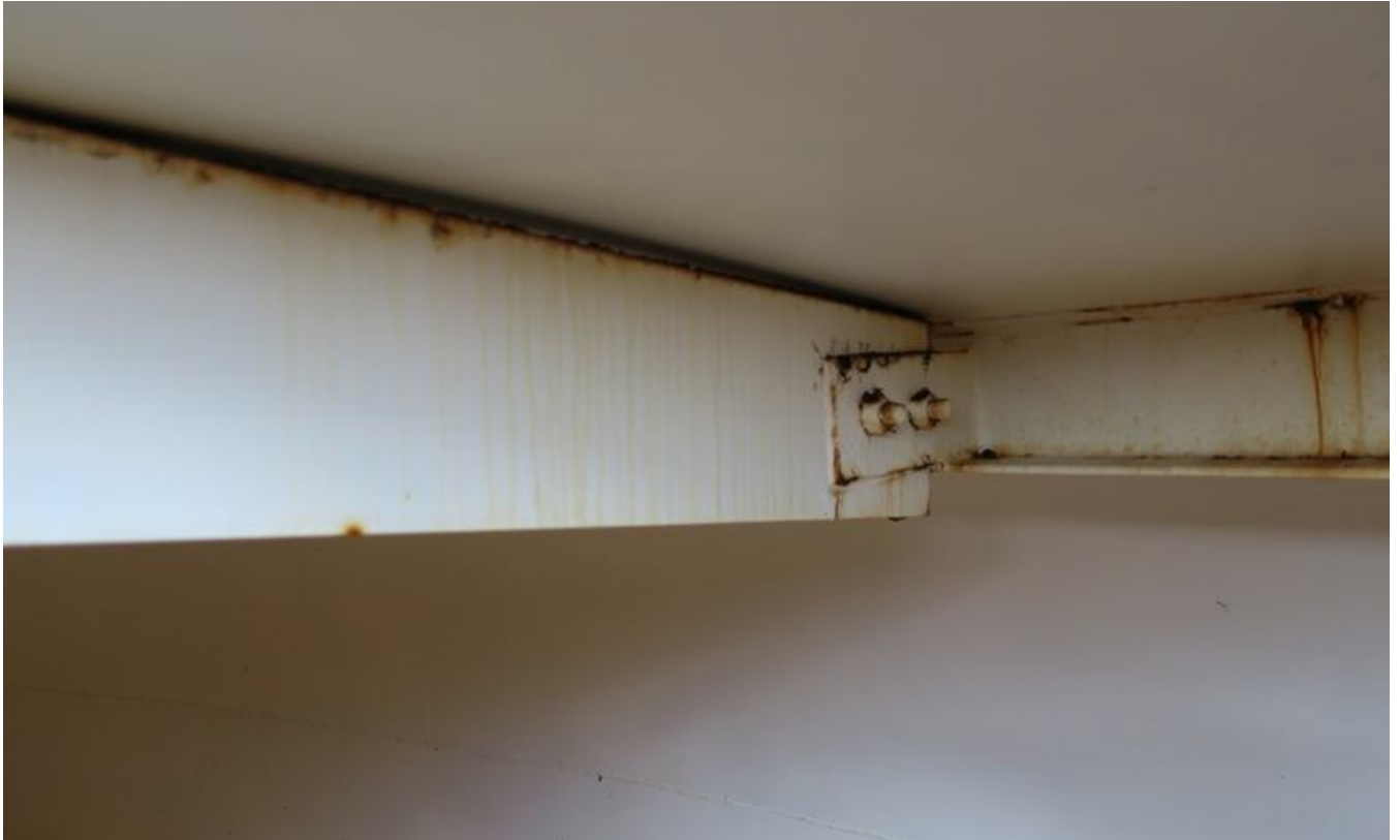
64. Rafter with bolted connections. Note corrosion.
