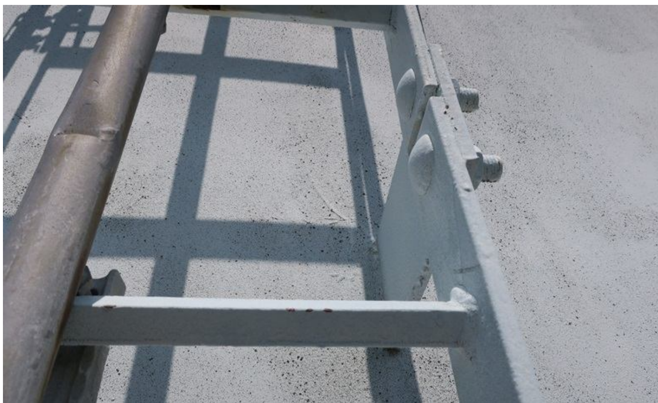
34. Exterior ladder connection.
