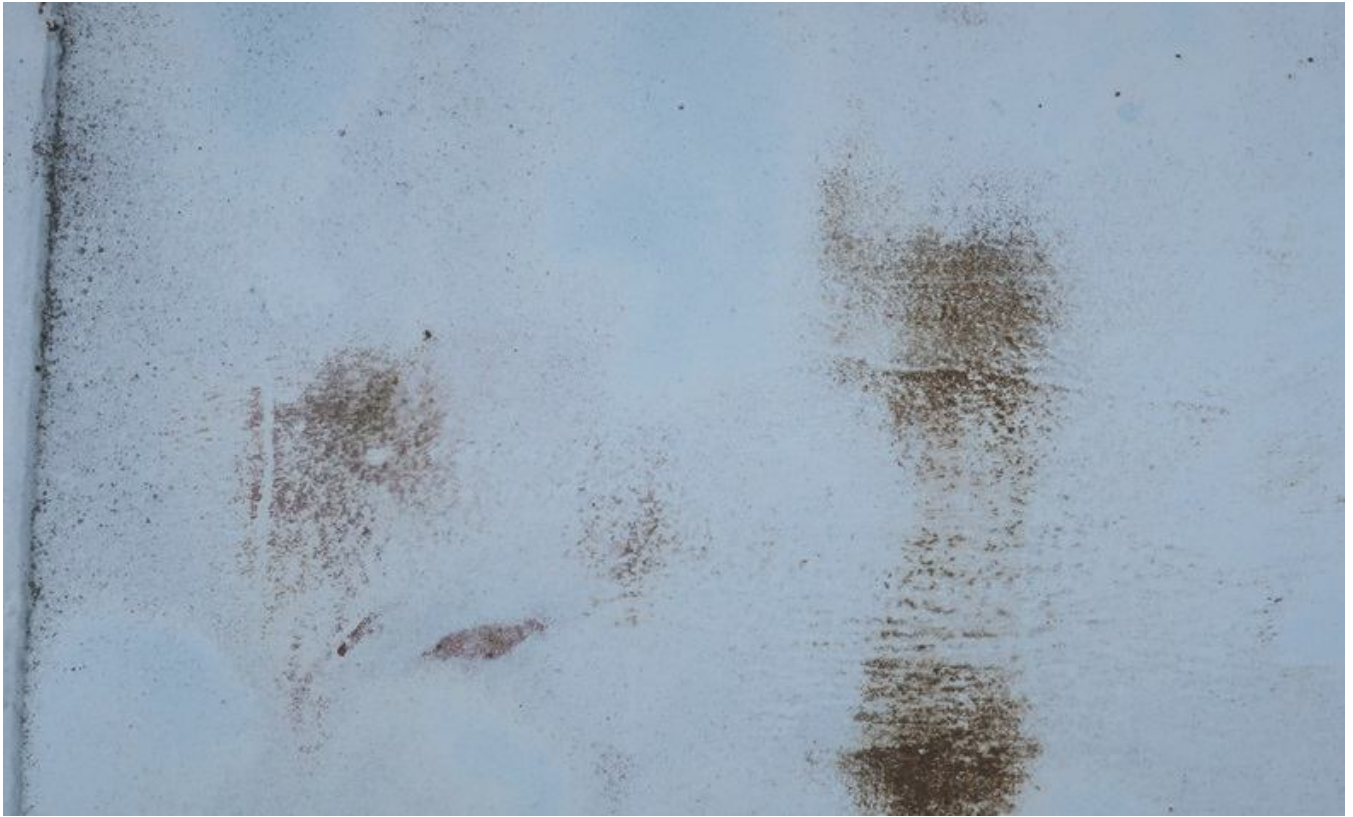
51. Roof corrosion.
