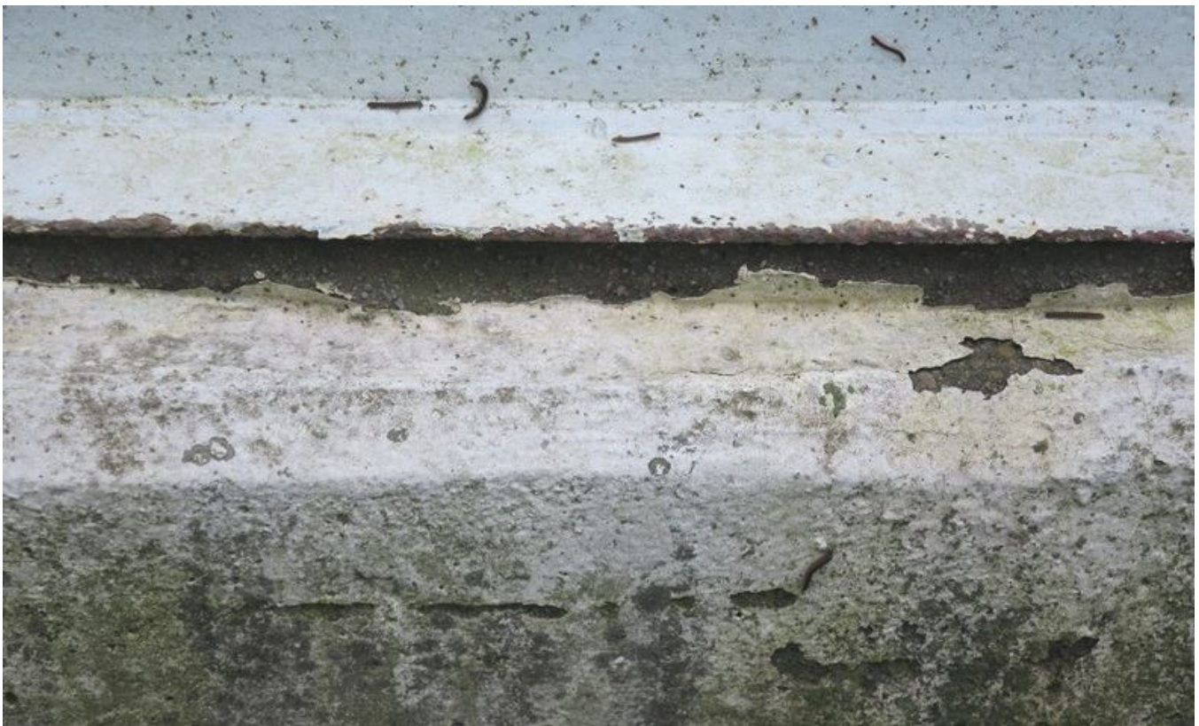
20. Tank foundation. Note coating cracking and chipping.
