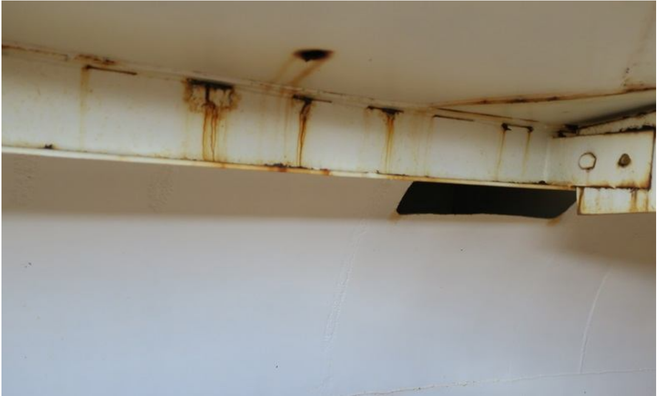
66. Support rafter and bolted connection. Note corrosion and missing bolt.
