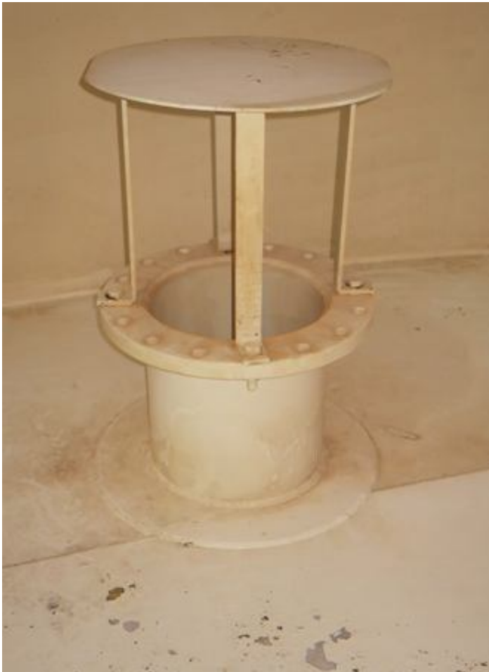
83. Blistered coating and corrosion on tank floor.
