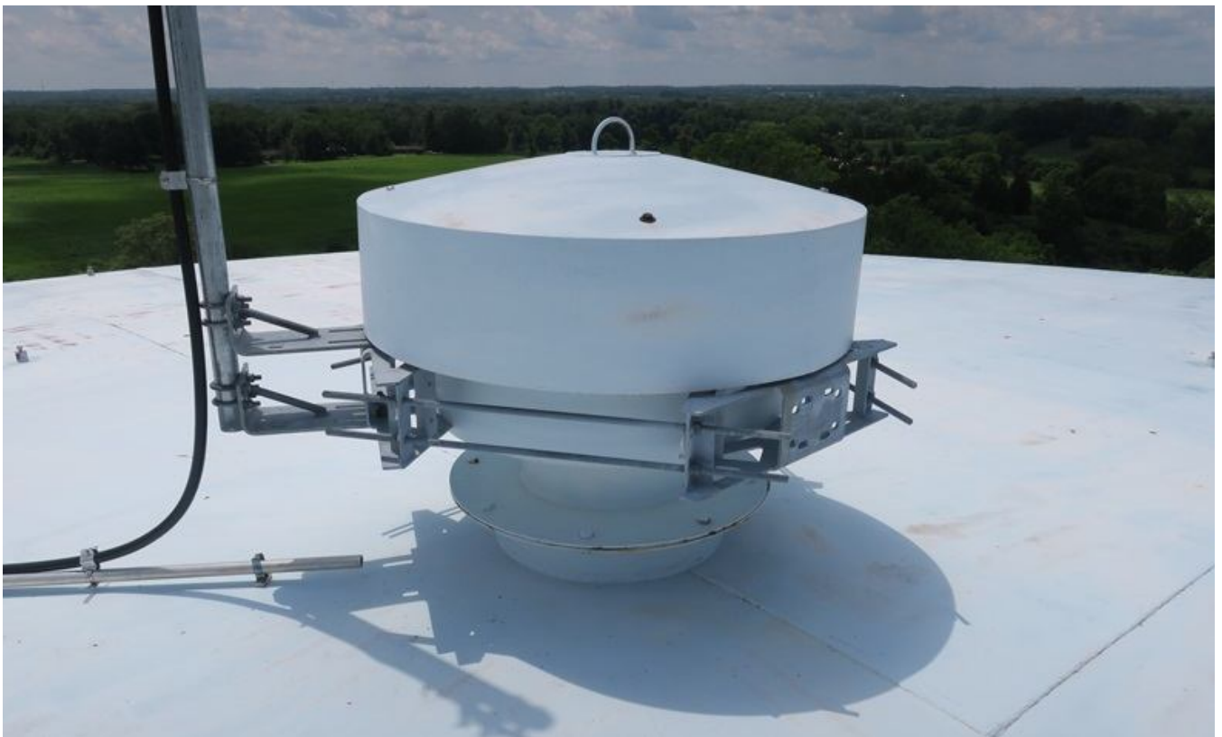
42. Roof vent and antenna. Note vent lug.
