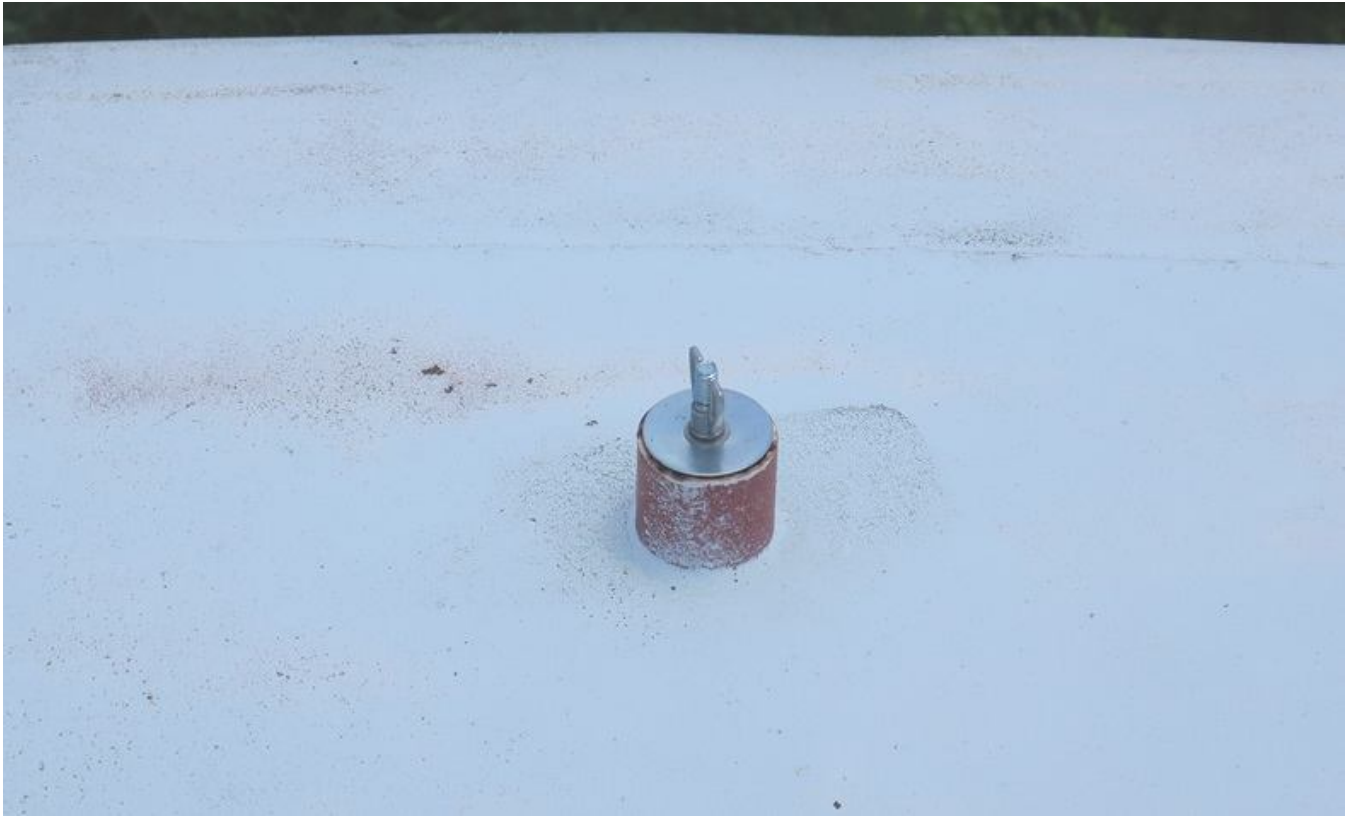
49. Roof plugged coupling.
