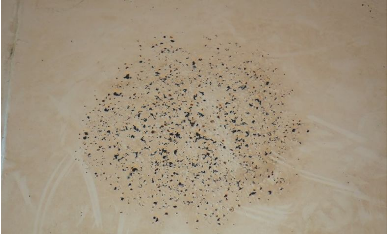
82. Blistered corrosion on coating and tank floor.
