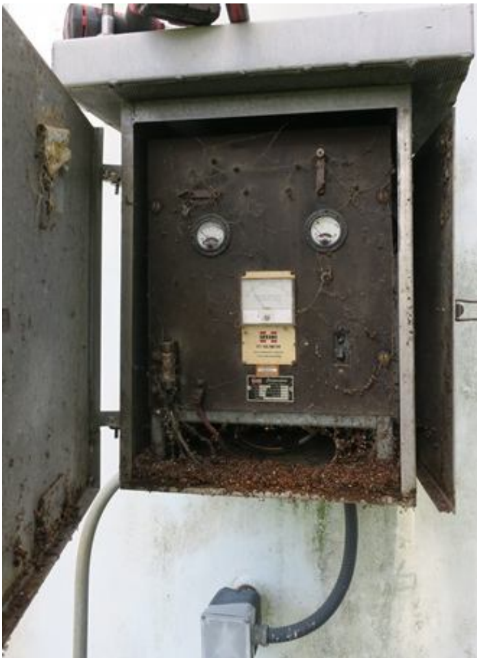
24. Cathodic protection cabinet.
