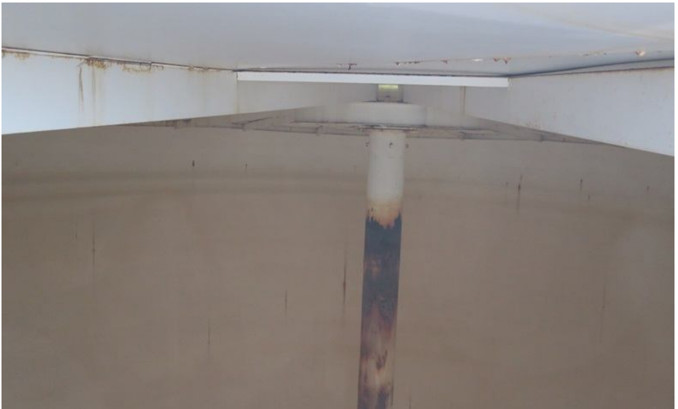
58. Interior roof, support column, and rafters.
