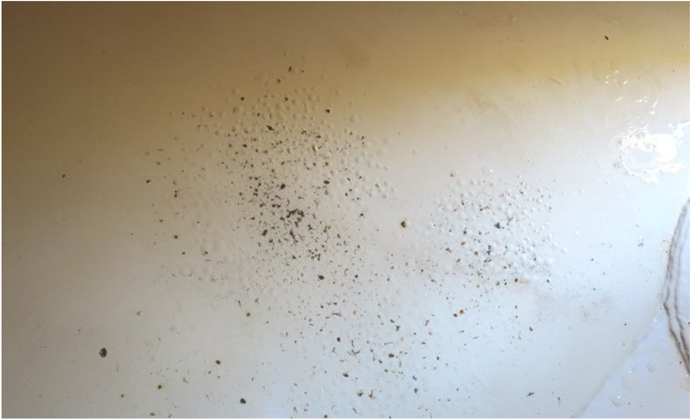
81. Blistered coating and corrosion on tank floor.
