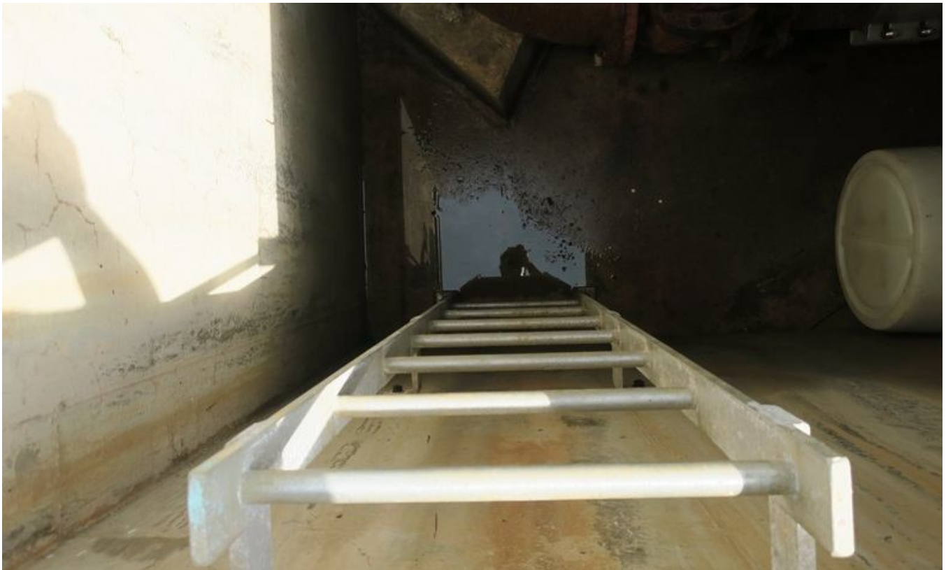
14. Valve vault ladder. Note standing water.
