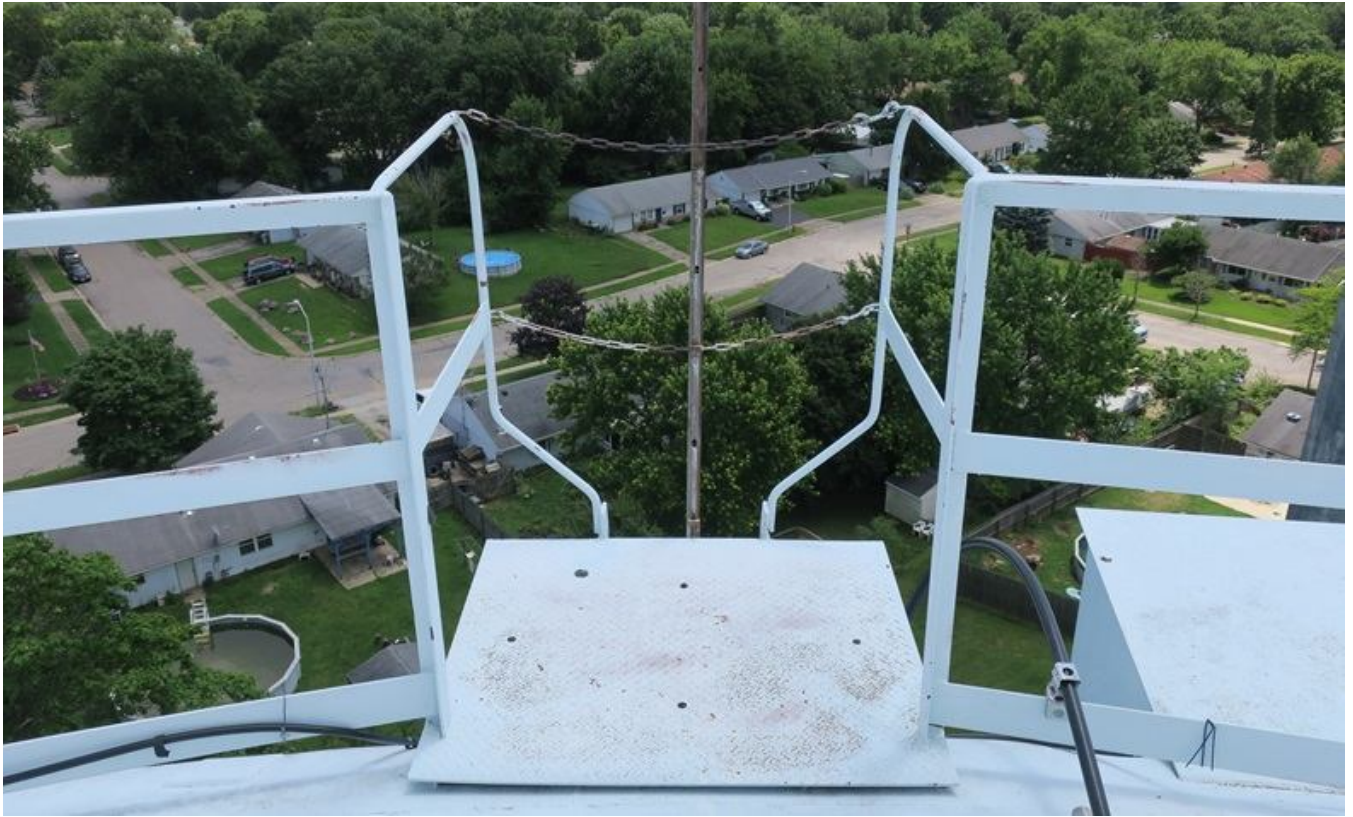
47. Roof access and safety railing. Note closure chains.
