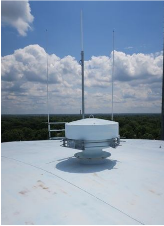
41. Roof vent and antenna.
