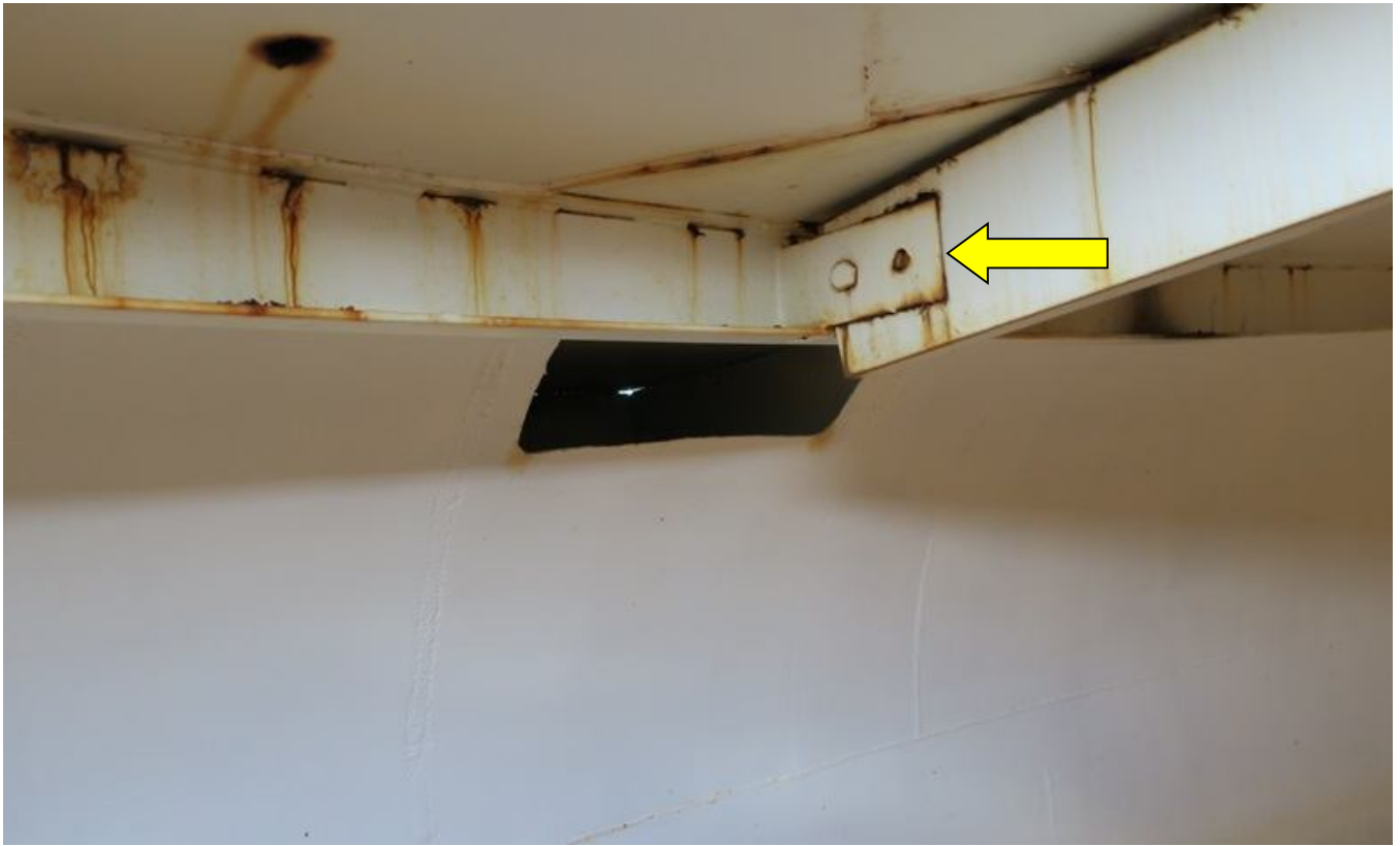
67. Rafter and bolted connection. Note corrosion, missing bolt, and overflow inlet.
