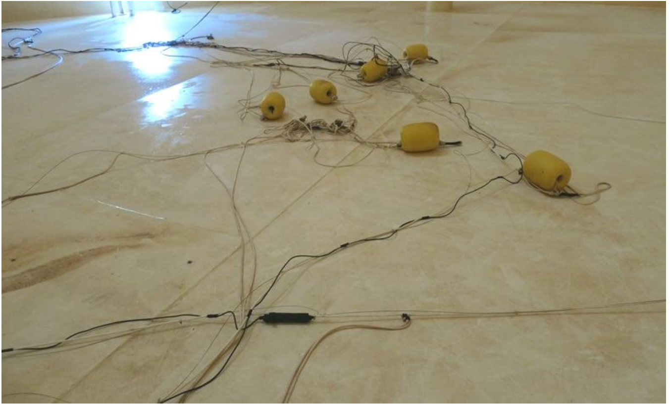
79. Cathodic protection equipment on floor.
