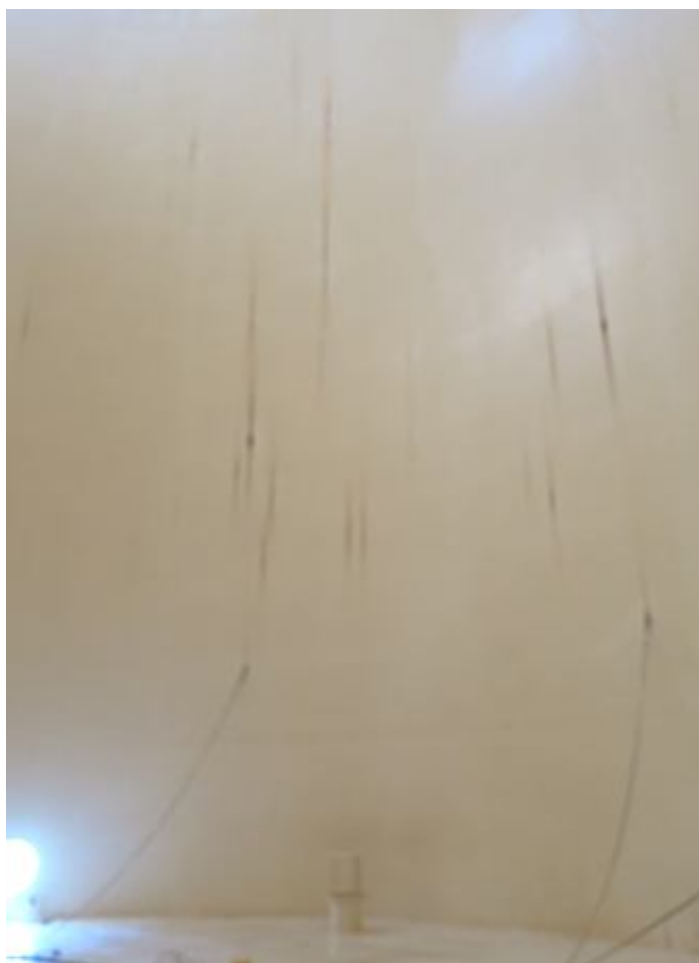
72. Tank interior. Note corrosion.
