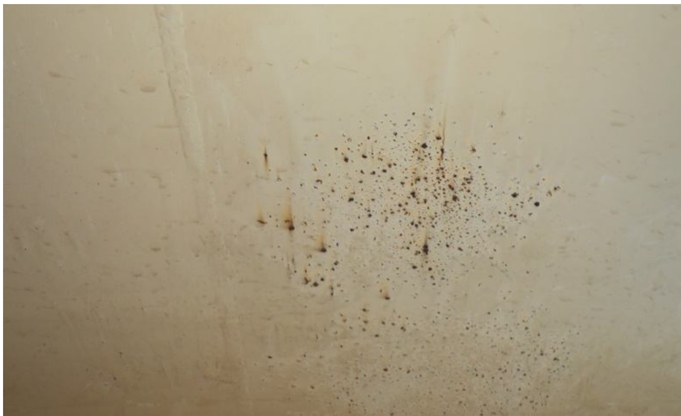
76. Blistered coating and corrosion on tank shell.
