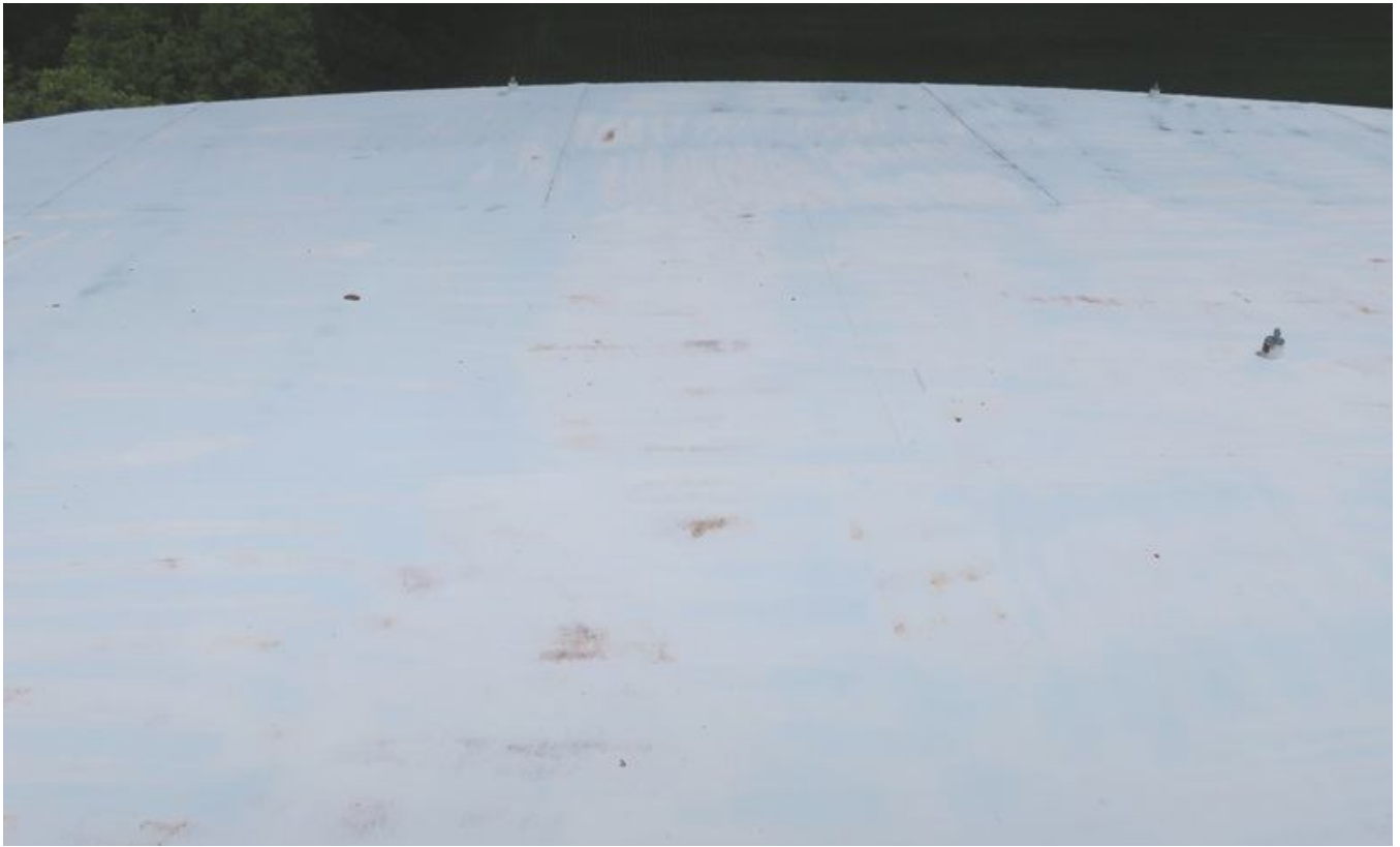
53. Roof corrosion and weathered coating.
