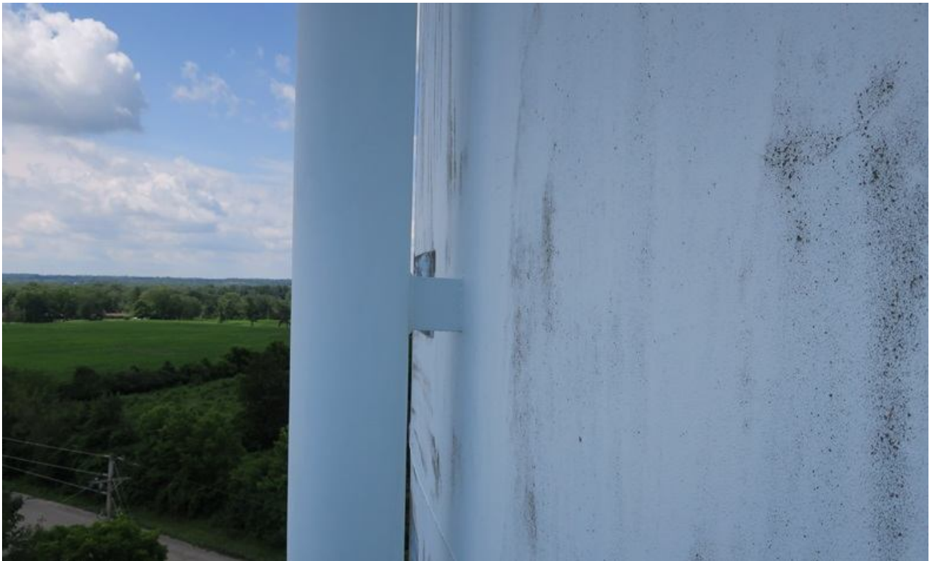
36. Overflow pipe bracket.
