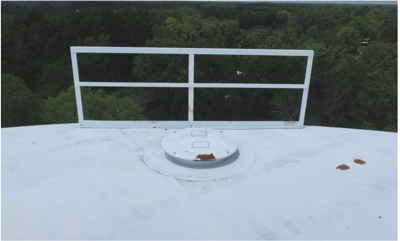
39. Roof manhole and safety railing.
