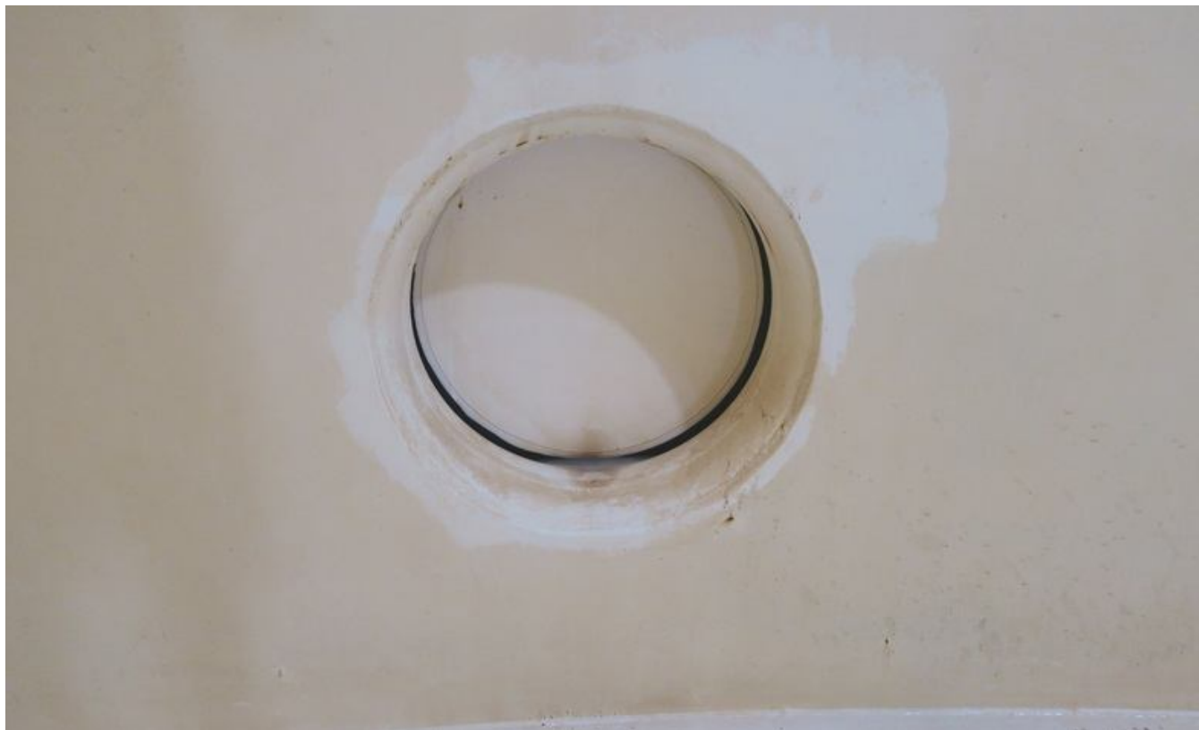
75. Shell manhole interior
