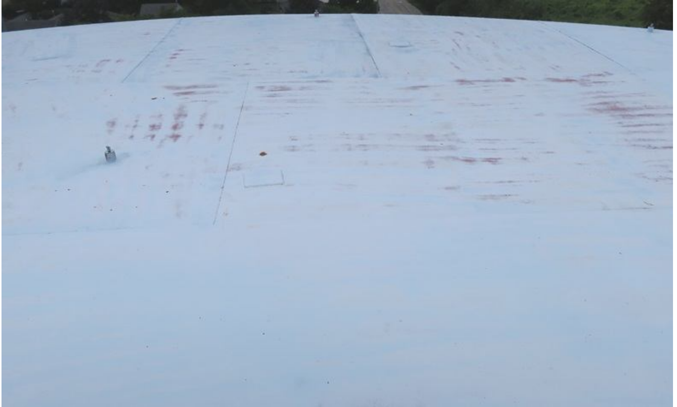
52. Weathered roof coating.
