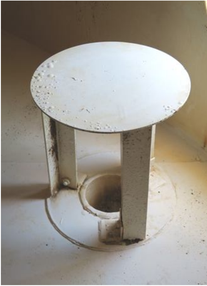
85. Drain pipe and removable cover.
