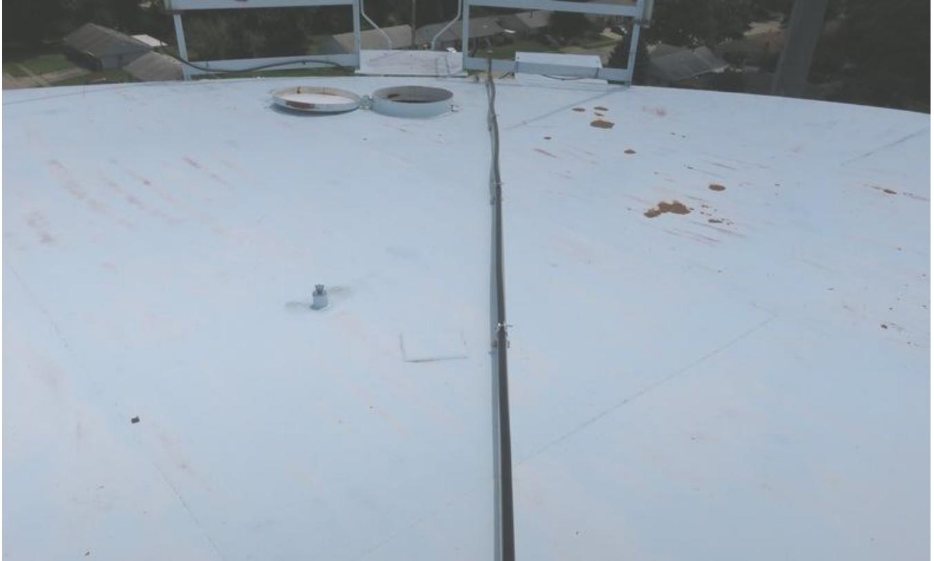
44. Roof antenna cable.
