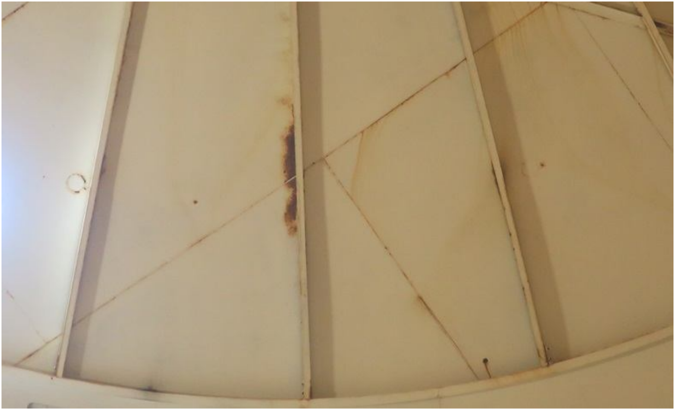
63. Corrosion on roof interior.
