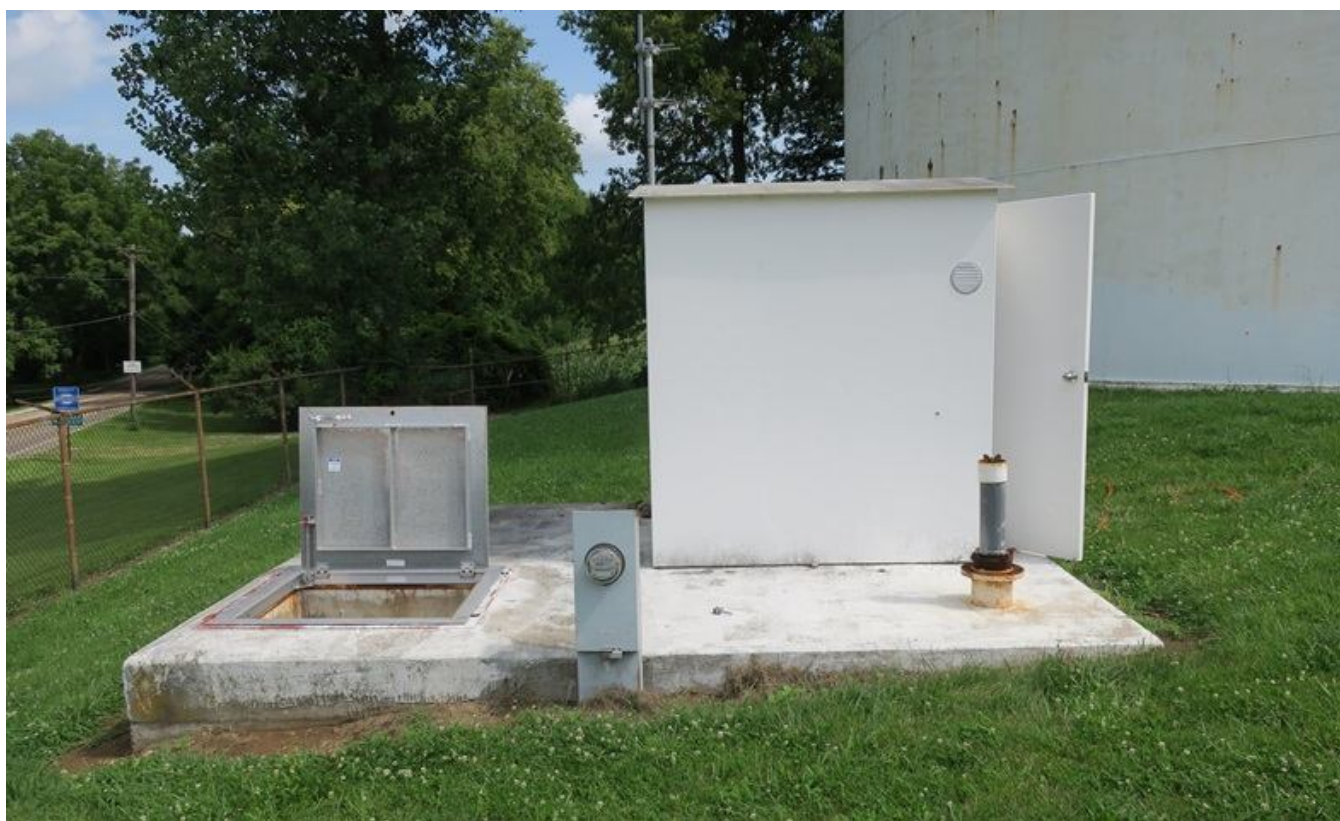
12. Valve vault access, shed, and electric meter.
