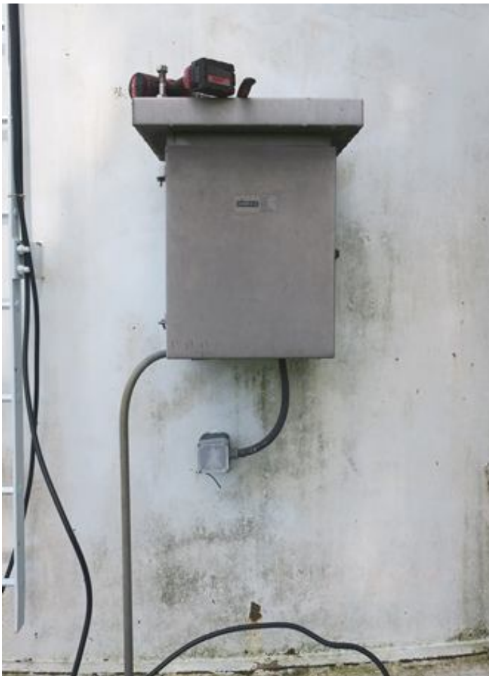
23. Cathodic protection cabinet.
