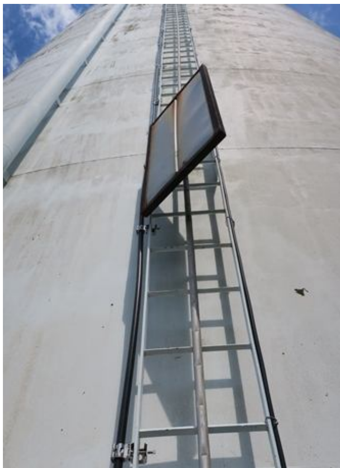
29. Shell exterior with spot corrosion.
