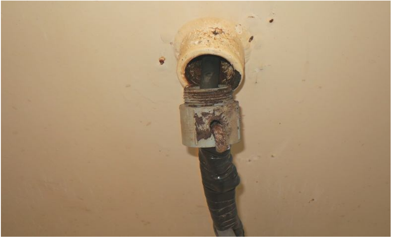
77. Broken cathodic protection equipment fitting.
