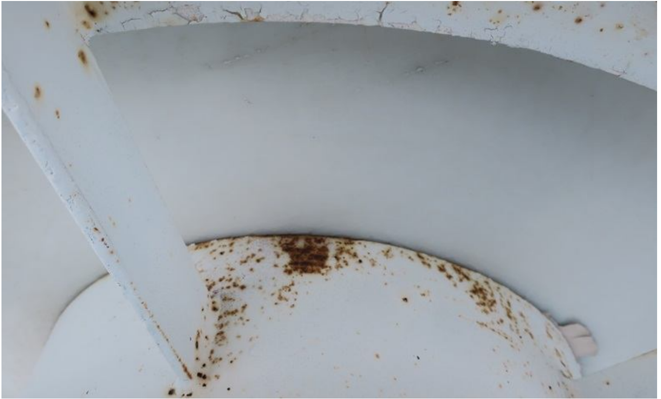
43. Roof vent. Note spot corrosion.
