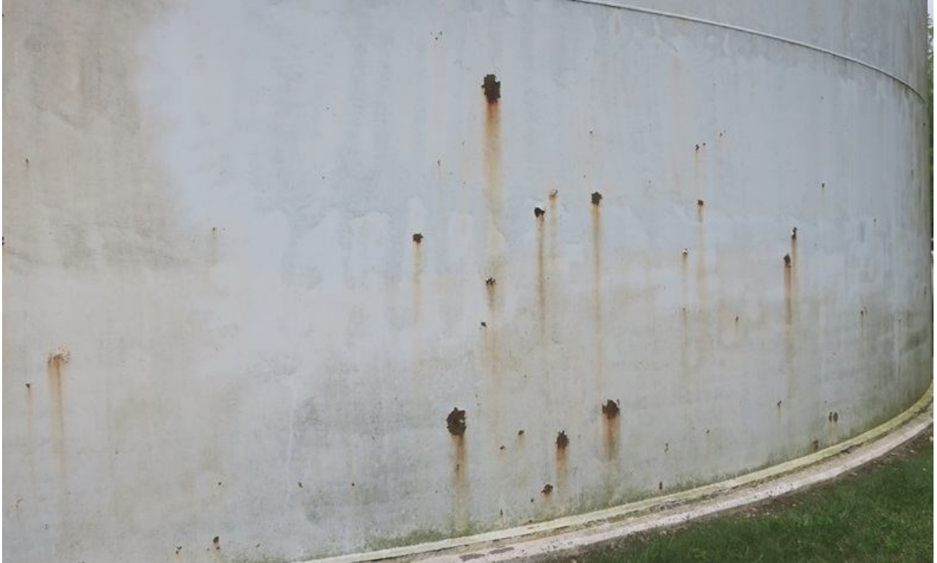
22. Shell exterior with spot corrosion.
