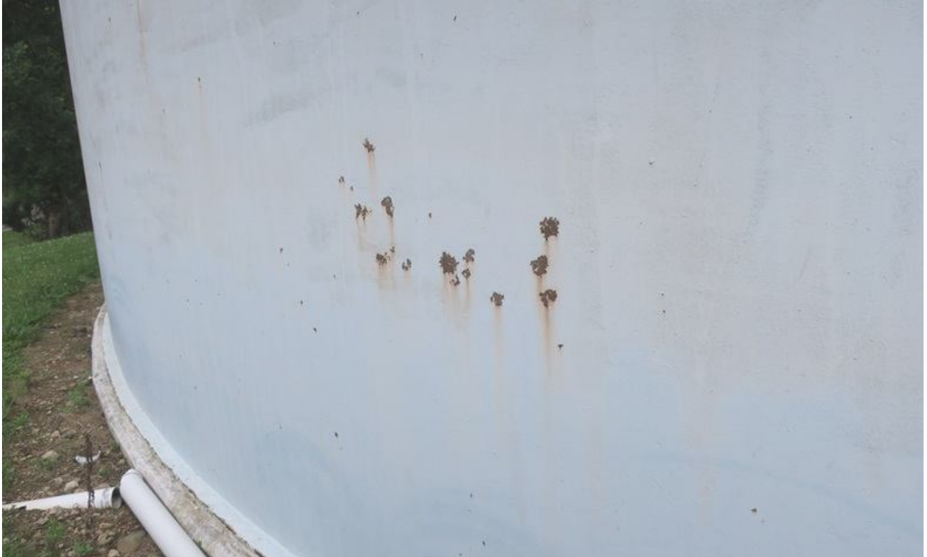
18. Shell exterior with spot corrosion.
