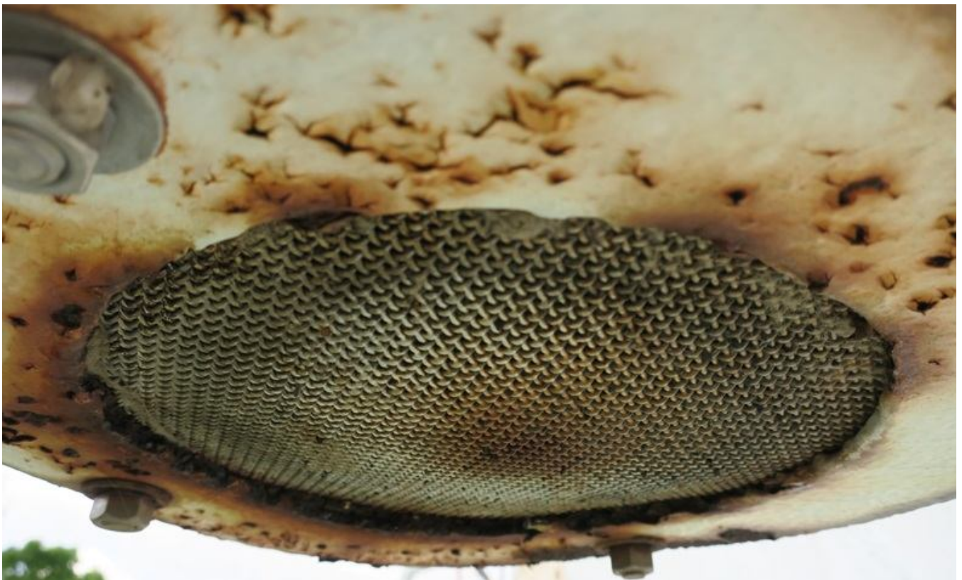
26. Overflow pipe drain. Note corrosion.
