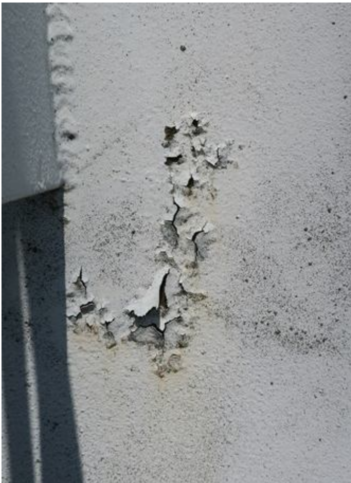
32. Paint failure along shell exterior.
