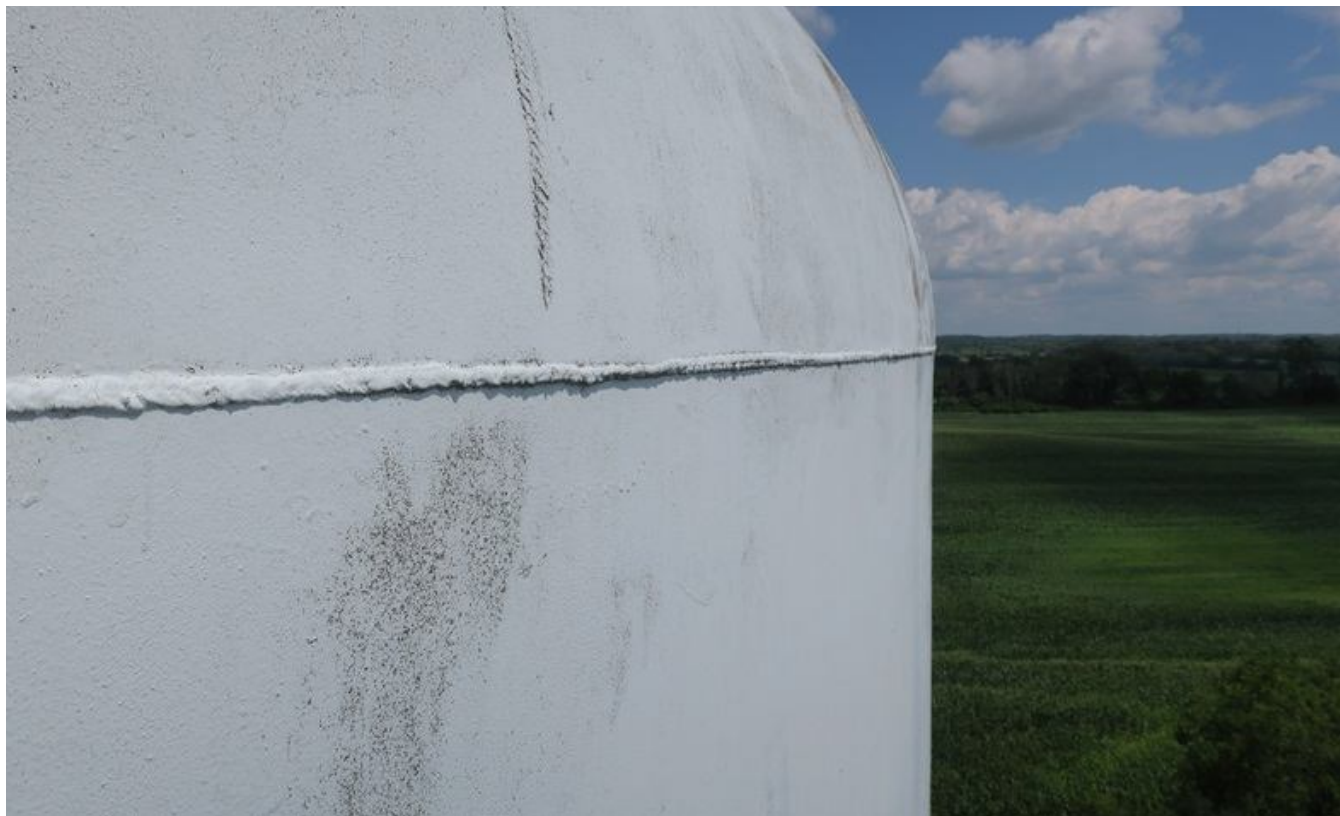
37. Shell exterior weld seam.
