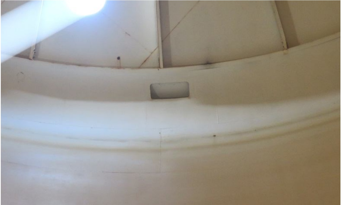
68. Overflow inlet and roof manhole opening.
