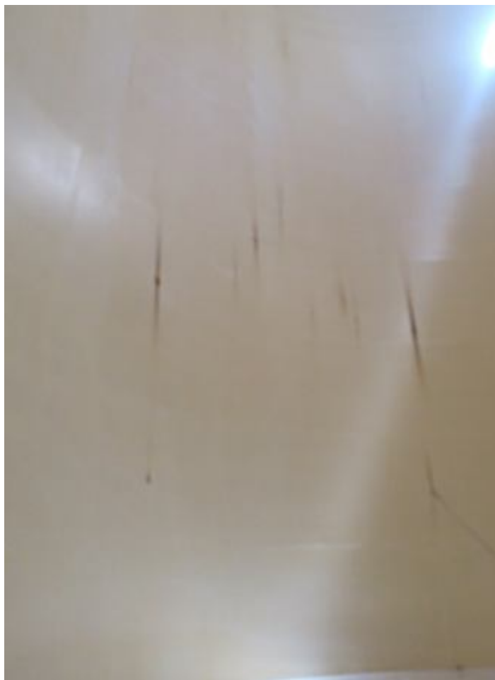
74. Tank interior. Note corrosion.
