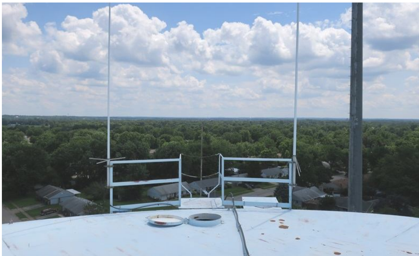
38. Roof access, platform, antennas, manhole, and safety railings.
