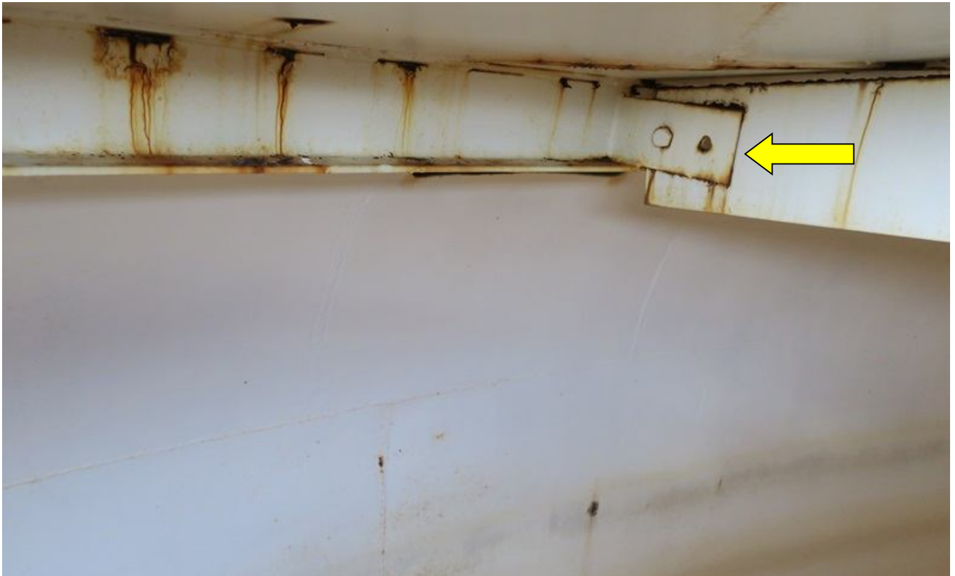
65. Rafter with bolted connections. Note corrosion and missing bolt.
