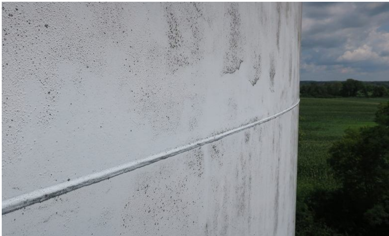
33. Shell exterior weld seam.
