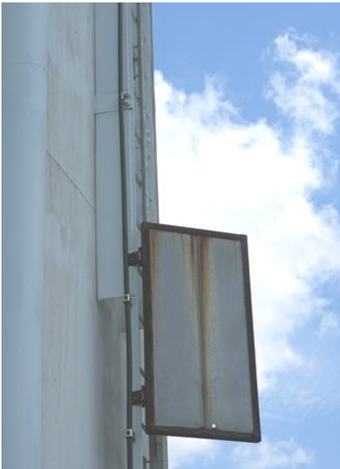
31. Exterior ladder and vandal deterrent.
