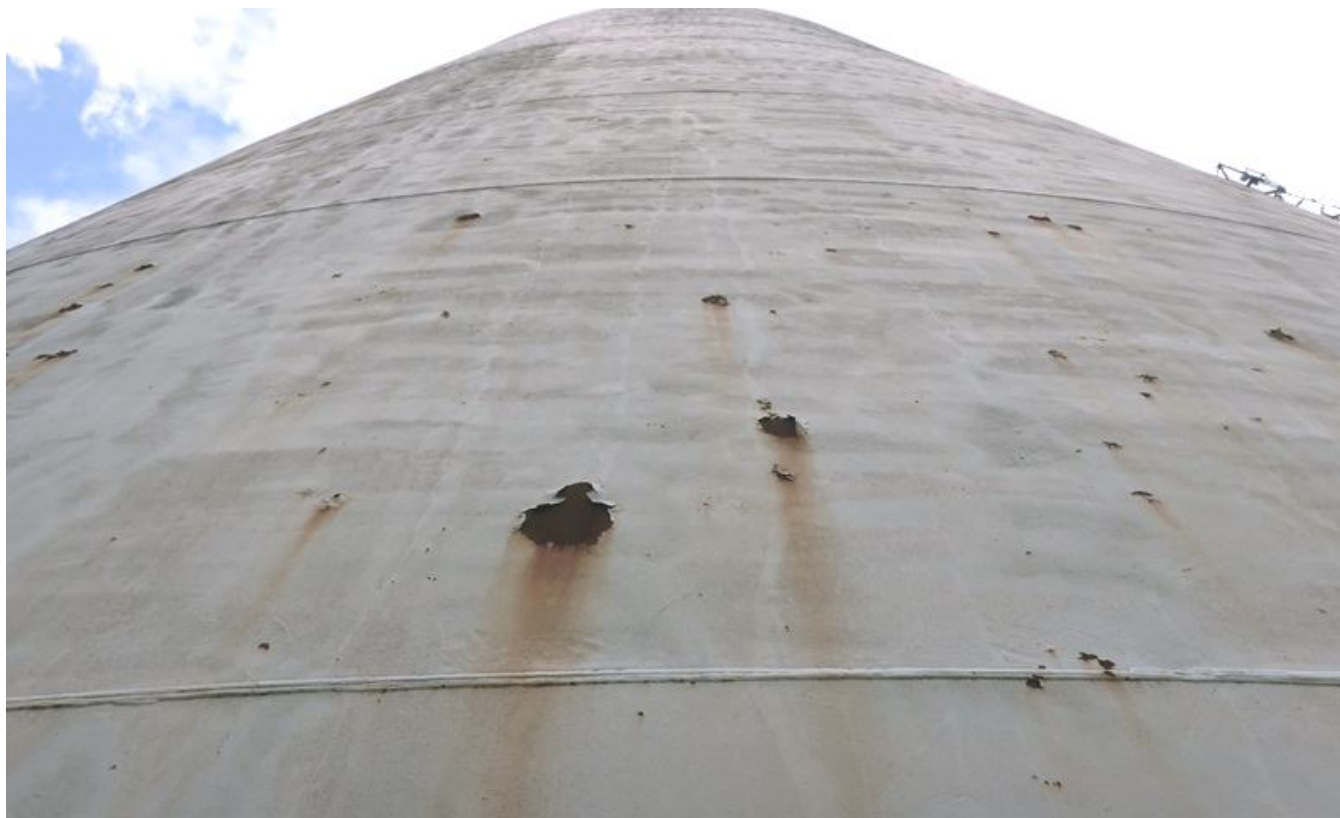
29. Shell exterior with spot corrosion.
