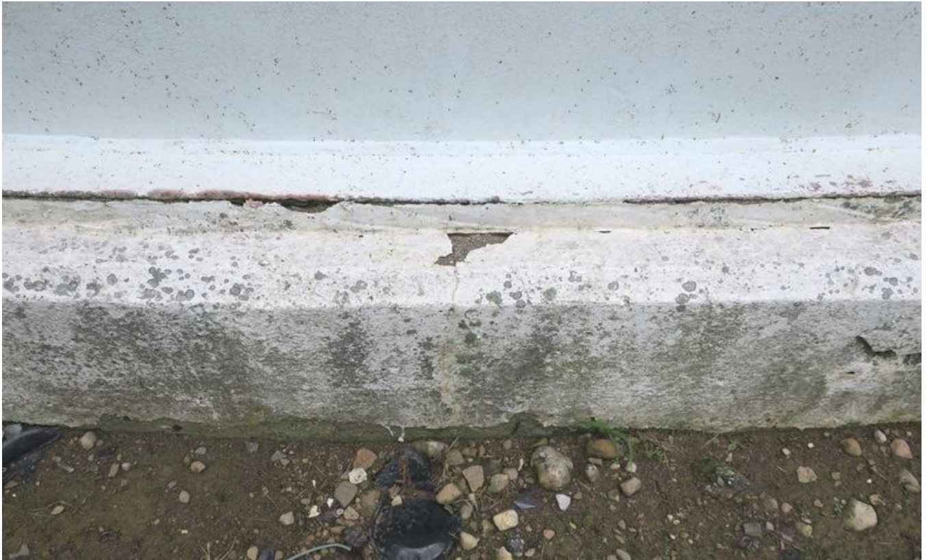
19. Tank foundation. Note coating cracking and chipping.
