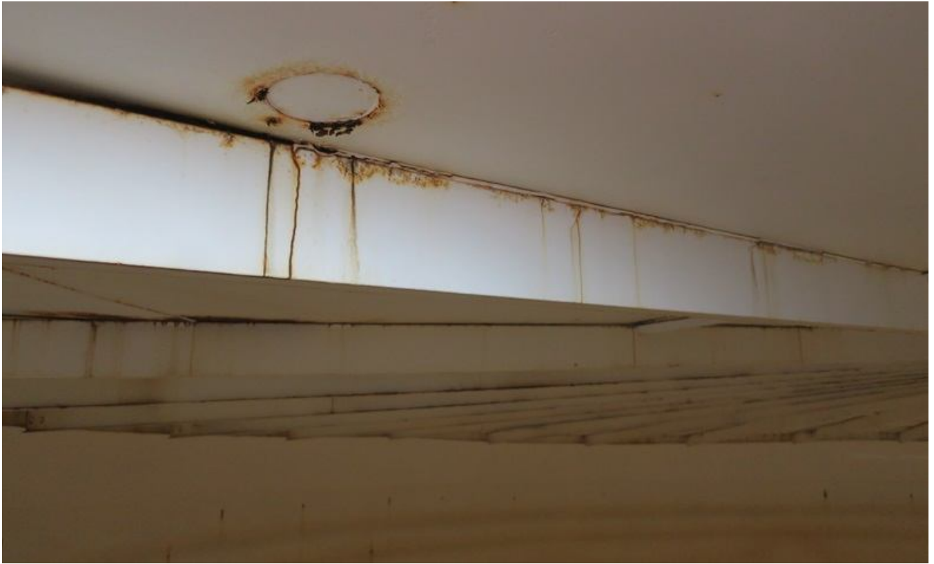
61. Support rafters. Note corrosion along rafters and circular welded patch plate.
