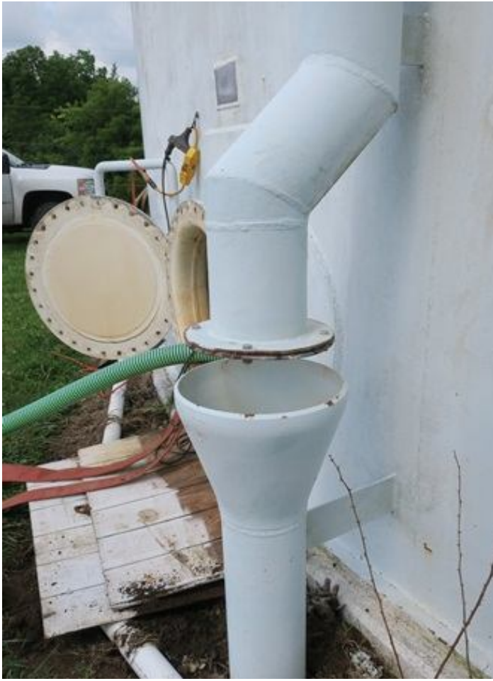
25. Overflow pipe air break and drain.
