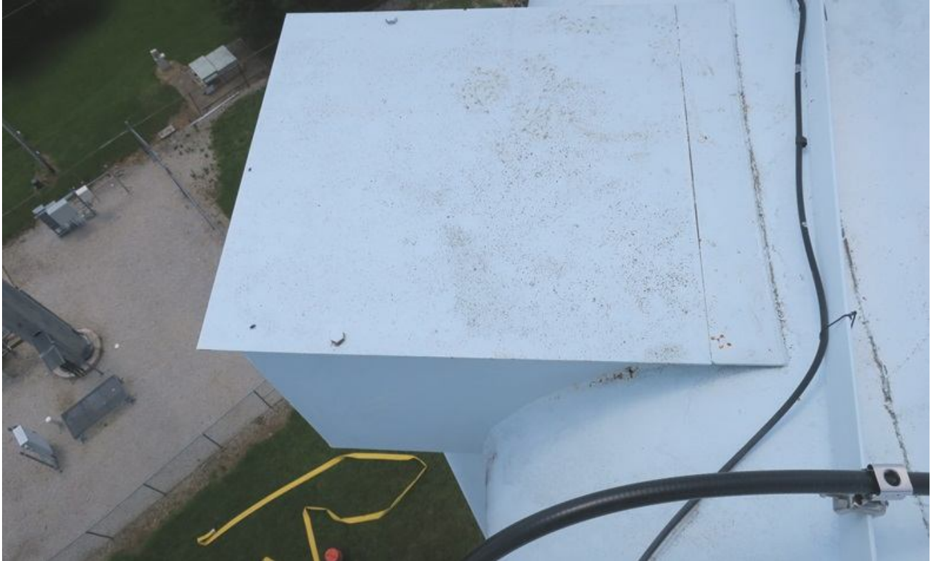
48. Exterior overflow weir box.
