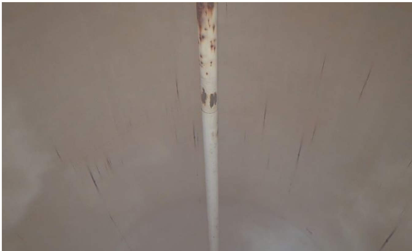
69. Tank interior and support column. Note corrosion along column.
