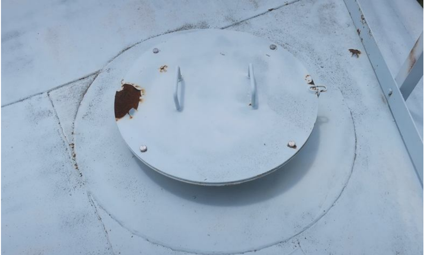
40. Corrosion on roof manhole cover.
