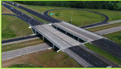
New bridge deck over US68 (photo courtesy of Michelle Porr)
